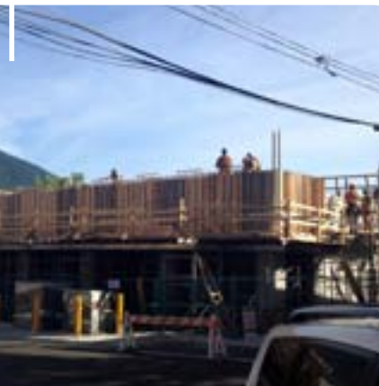
Pouring the concrete floor of the Co-op's new store.
